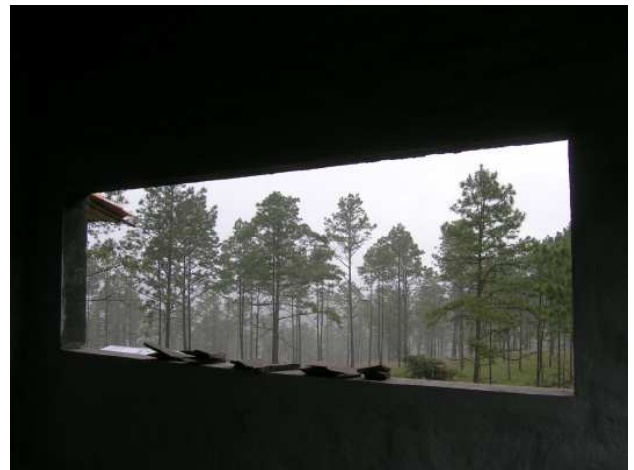
View from the second floor window of the rehab center
